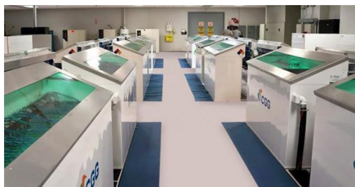
Picture 2 : Example of Immersion data center
